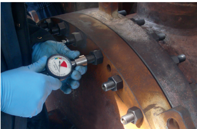
RT-Bolt load measurement underway during assembly of an exchanger channel cover with 3/4" diameter bolts
